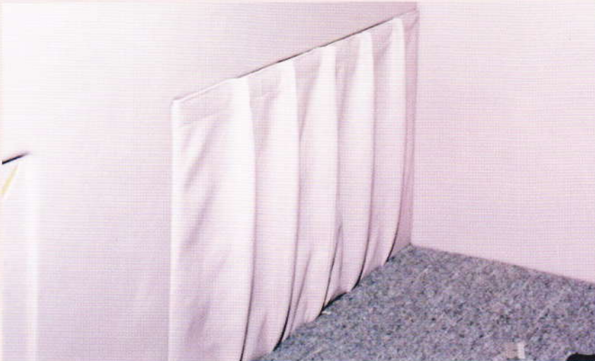
Photo 17. This is the exit area of the elastic. Frank will pull it snug then staple it to the panel. Don't make the elastic too tight. It will overstretch when the pocket is opened and tear away from the panel.
